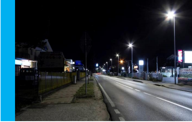
After installation of Grah LSL® 60
